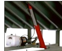
Fully Hydraulic Yieldable Lip Cylinder
