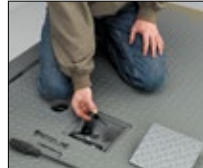
Maintenance inspection plate in the deck to allow for maintenance above the dock.
